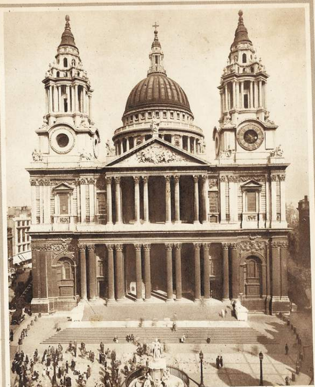
St. Paul's Cathedral, London, which has been referred to as the "Parish Church of the Empire." It stands in the heart of the City and is the third, if not the fourth, cathedral to occupy the site. In Cromwell's days eight hundred horse were stabled within the building of that time, which was destroyed in the Great Fire. The present edifice was designed and built by Sir Christopher Wren, his great work ending in 1710. The top of the Cross on the dome is 365 feet above the pavement.
